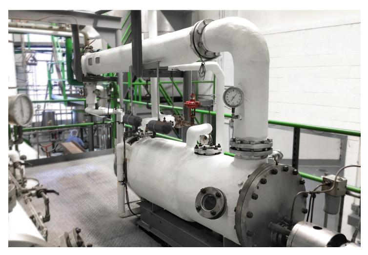
We have 5 distillation units, but out largest production unit is an all stainless steel, two column, continuous still. The feed rate is up to 500 lbs/hr for dry vacuum distillation.
